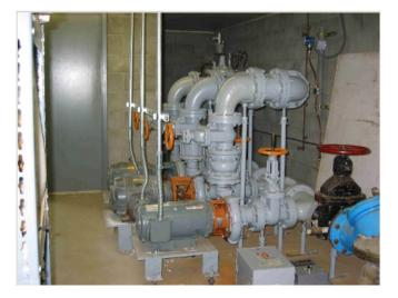
The faulty motor is being controlled by a VFD. There is an external Disconnect Switch located adjacent to the VFD.
